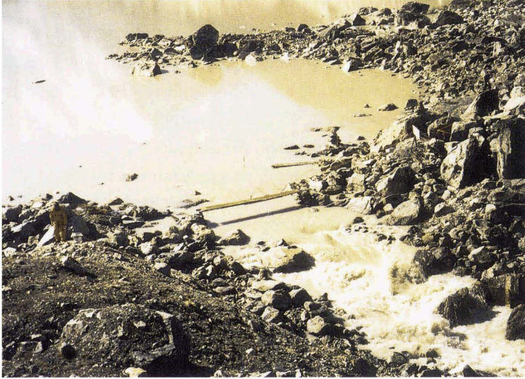
Photo 33 : Overlooking view of the outlet. Level gauge being installed near a bridge temporarily constructed.
